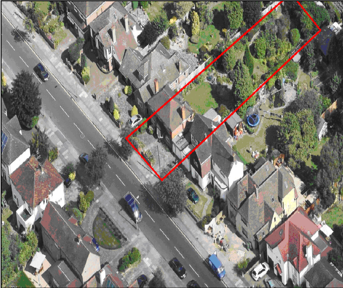
Existing aerial view.
